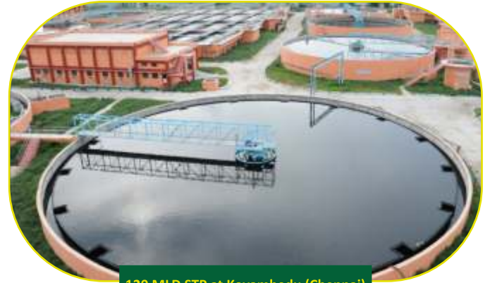
120 MLD STP at Koyambedu (Chennai)
